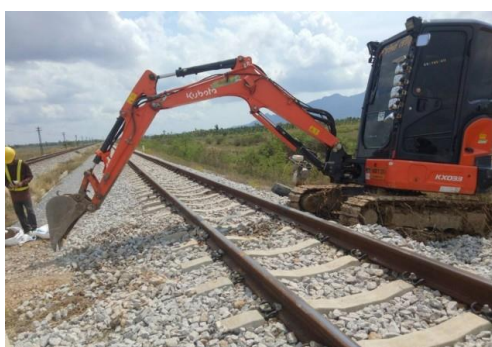
Installation of Cable Trench and Laying Cable
