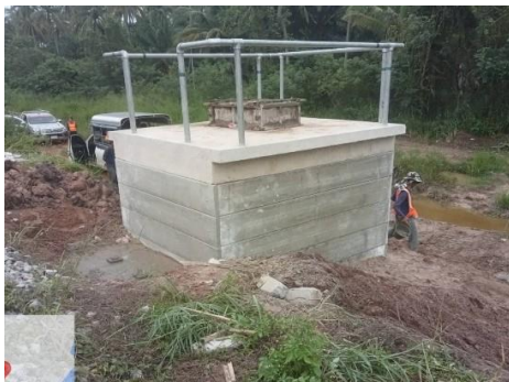
Construction of Concrete Foundation of LOC and Signal
