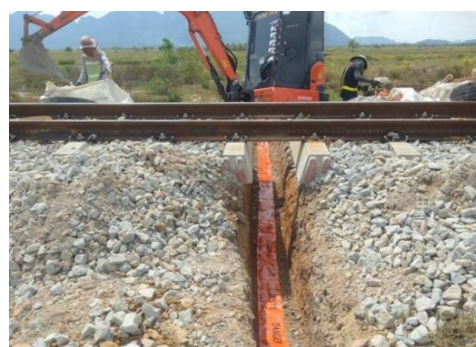
Installation of Cable Trench and Laying Cable
