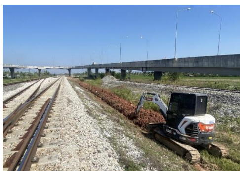
Installation of Cable Trench and Laying Cable
