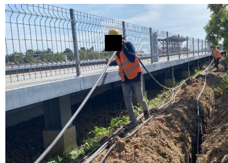
Construction of Cable Trench Bridge and Box Culvert
