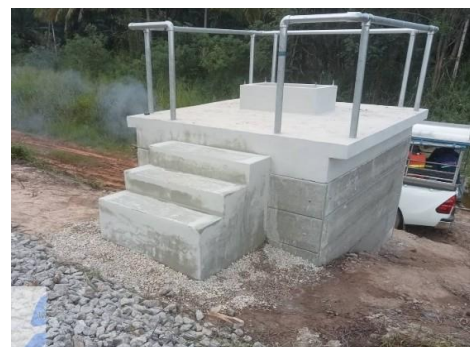
Construction of Concrete Foundation of LOC and Signal
