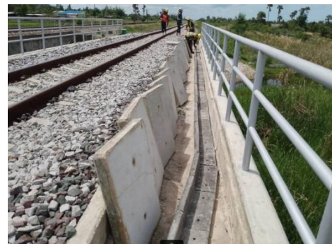
Construction of Concrete Foundation of LOC and Signal
